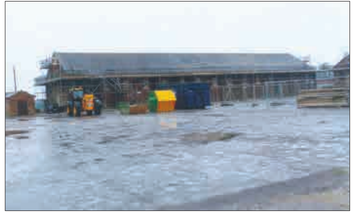
Work started on building P
